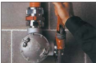
5. Install hub on enclosure
