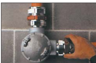
6. Insert cable and tighten red union
